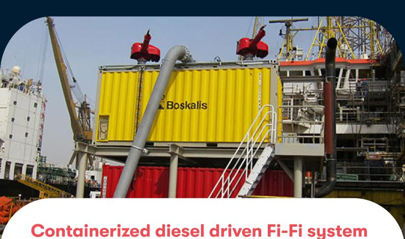
Dutch dredging contractor and marine services provider Boskalis has won the contract for a multi year charter of one of her Platform Supply Vessels (PSV) in the Middle-East. For this contract the vessel needed to be equipped with external fire fighting capability. For this project, Fischcon delivered a containerized diesel driven fire water pump set for
